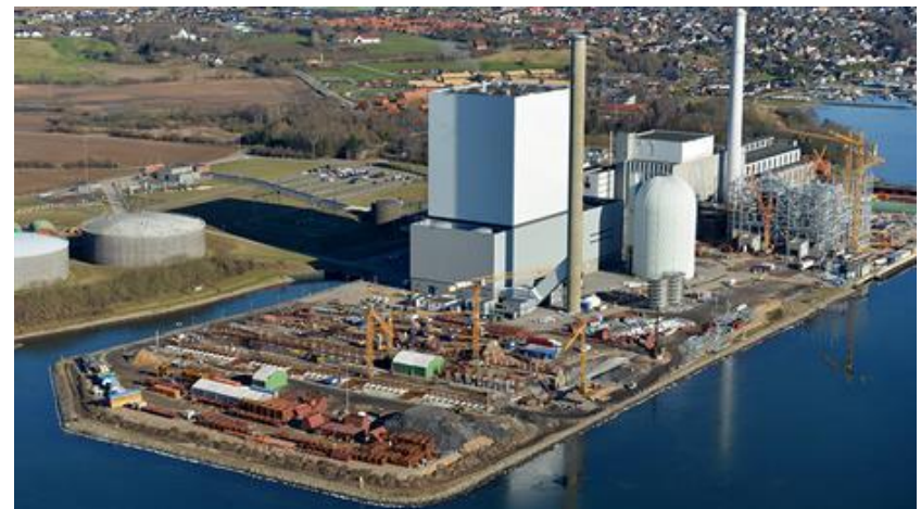
Start of construction 2015
