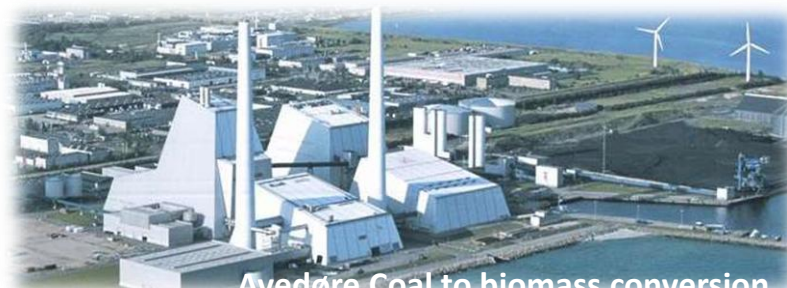
Avedøre Coal to biomass conversion
